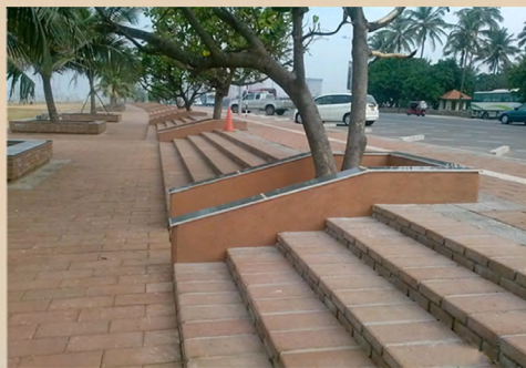
After the Project
