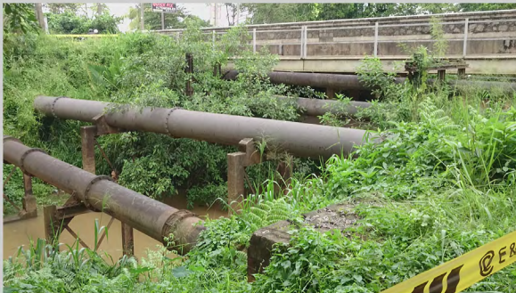
Near The Bridge
