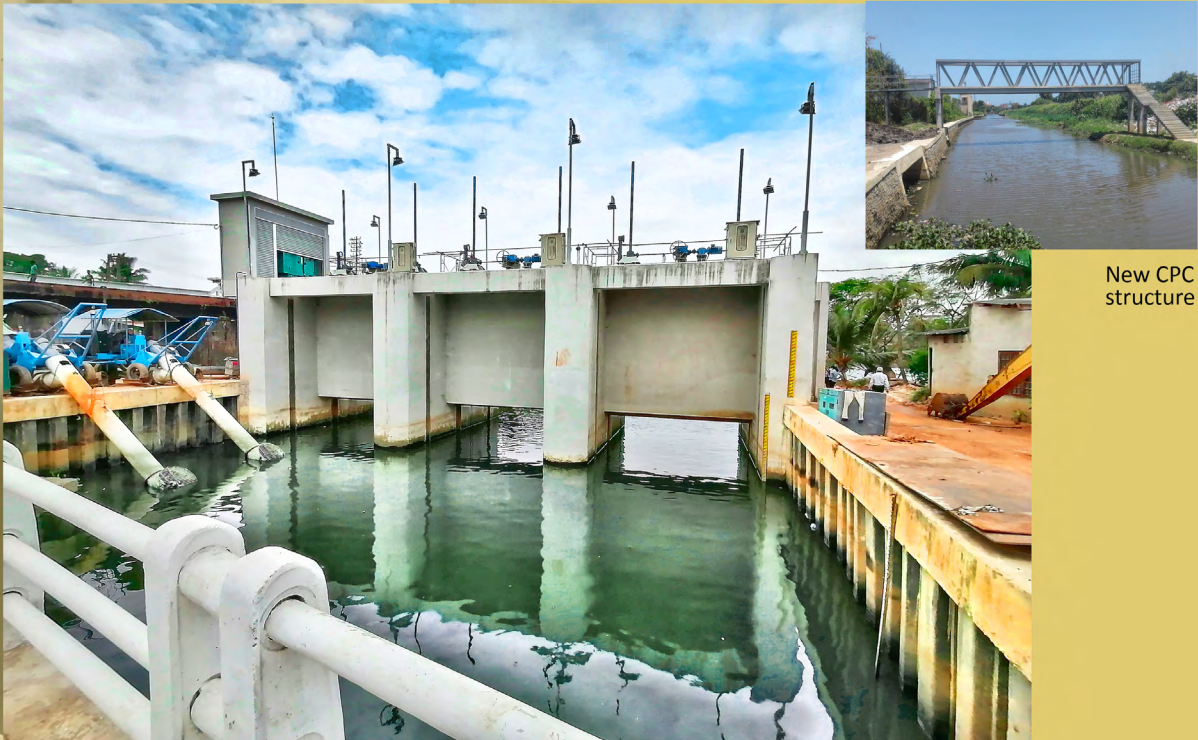
Flood gate structure at Kittampahuwa canal connection to Kelani River
