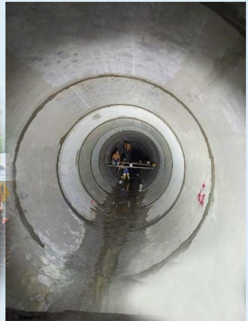
Torrington main Tunnel
