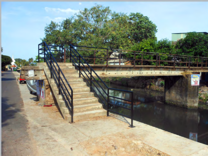
After the Project
